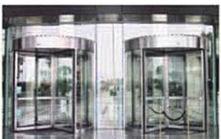
Shanghai Bank of China Tower
