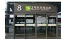
Shanghai Hongqiao International Airport
