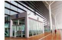
Tianjin Binhai International Airport
